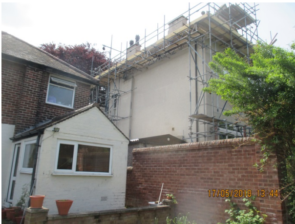
Looking west towards no. 3.
