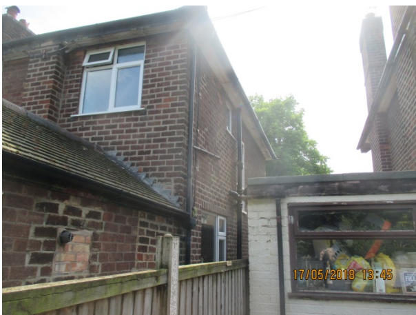
Looking south west towards boundary with no. 7.
